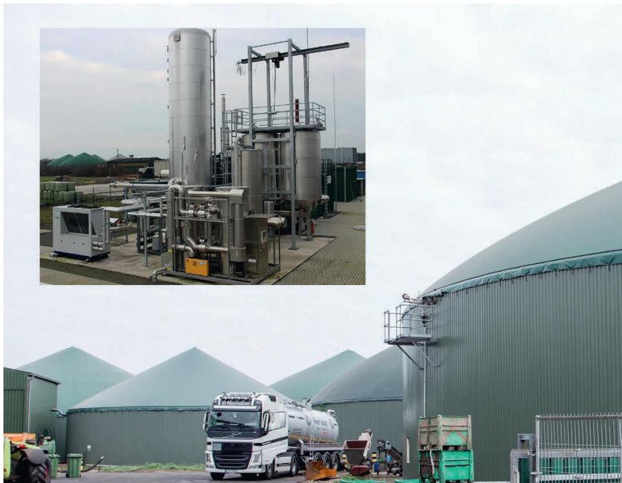
The amine scrubbing system has been proving as a reliable upgrading system
